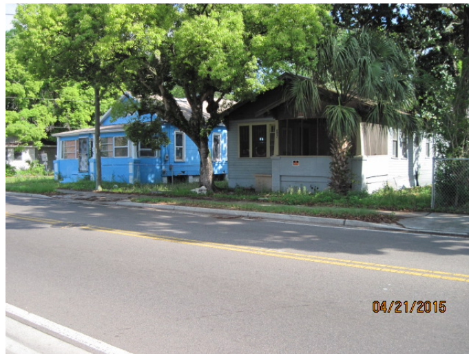
Residential uses across Golfair Boulevard
