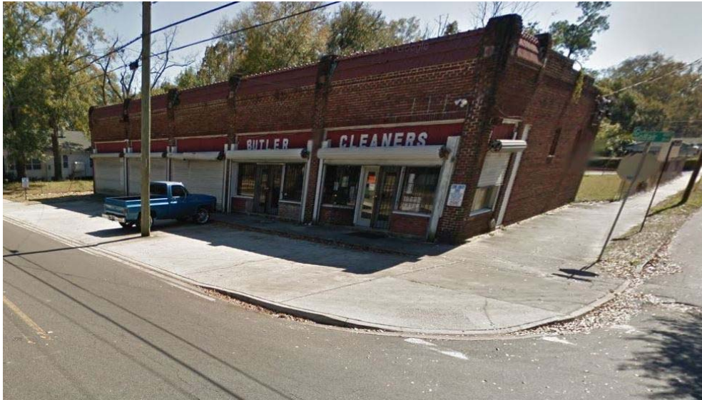
Existing Conditions Building frontage/ Source: Google Maps
